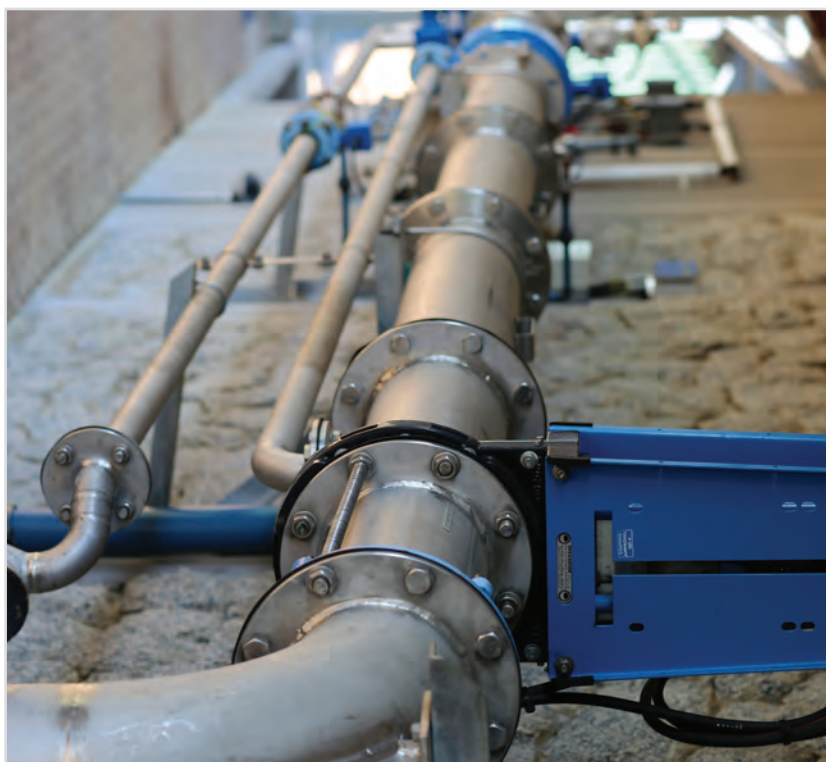
Stainless steel pipe in the Western Cape resists aggressive acidic soil conditions.
