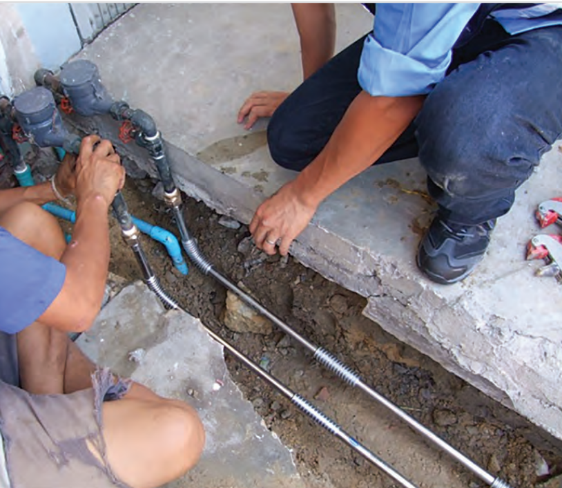
Corrugated pipe installation.
