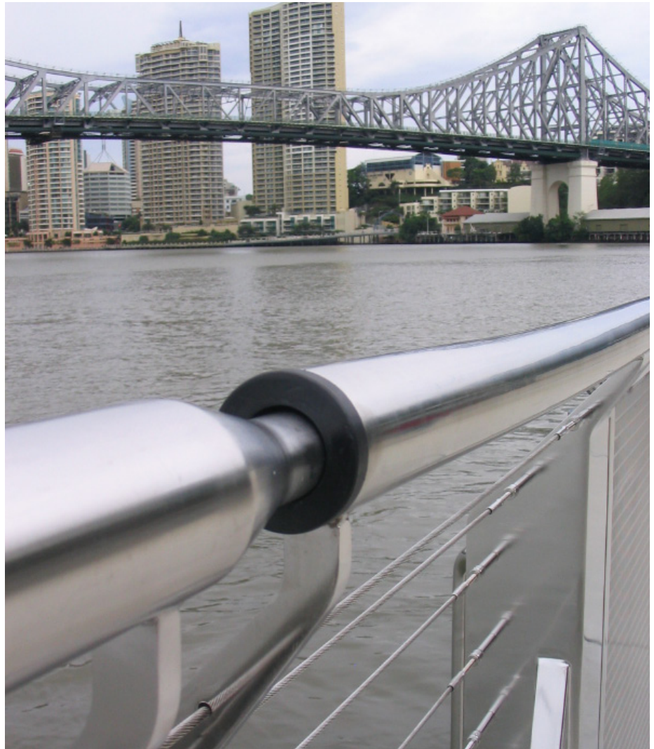
FIGURE 1: The floating walkway in Brisbane is an example of successful use of stainless steel in a marine environment.
